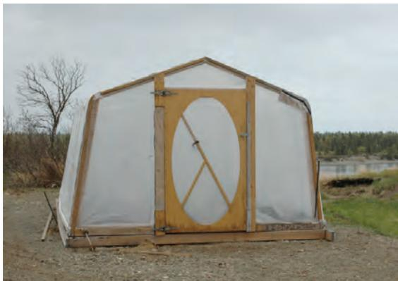
one of the commercial kits, the widths range from 10 ft to 35 ft. The most common lengths are 24 ft, 48 ft and 96 ft, but most kits can be ordered in any length you desire (in 4-ft increments). Before getting the structural kit for a custom-sized hoop house, make sure that you are able to get the greenhouse covering plastic for the proposed size.
